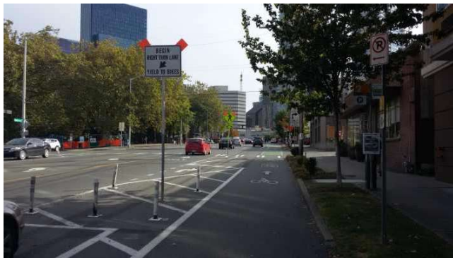
Figure 2: Mixing zone, Dexter Ave, Seattle
